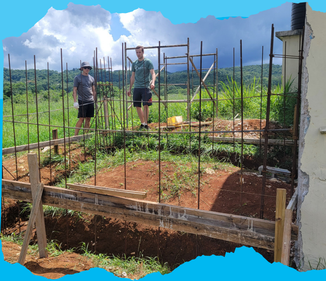
Here they are building a footer for a new shower room.
